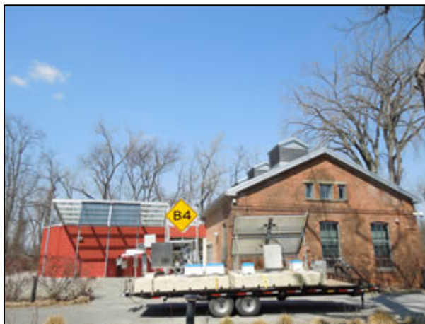
View of the Center for Environmental Innovation and Education with REON "B4" platform.
